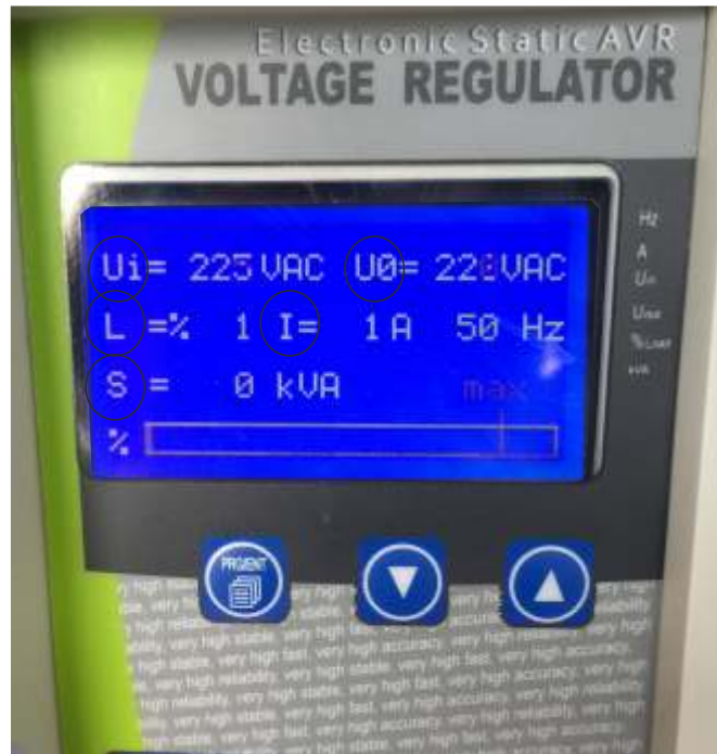
Figure 3.1 SVR Front Panel
